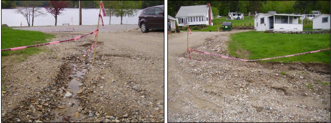
Figure 2: Two photos of the erosion prior to the paving improvements in the Newfound Sands Condominium Association roads. The photo on the left looks down to the lake, the photo on the right faces the opposite direction.
