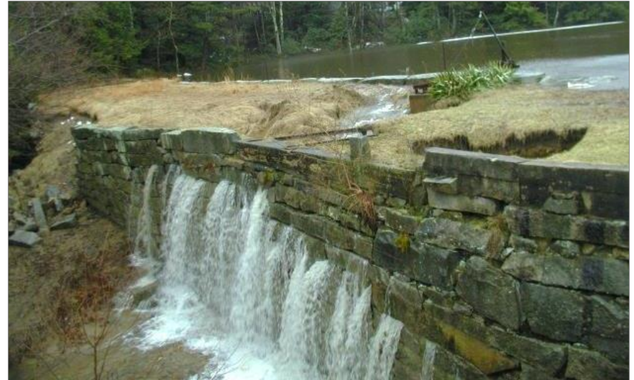
Breach at Haydens Mill Pond Dam, Hollis (Source: NHDES Dam Bureau)
