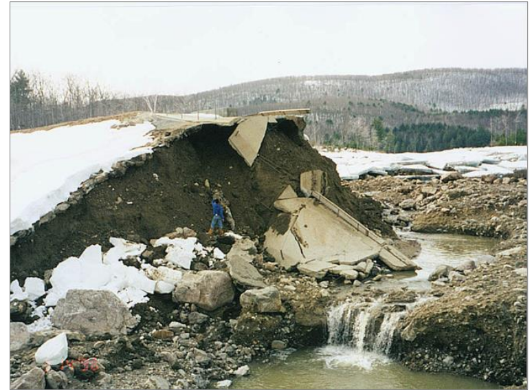
Breach at Meadow Pond Dam in Alton, March 1996 (Source: NH Department of Environmental Services, Dam Bureau)
